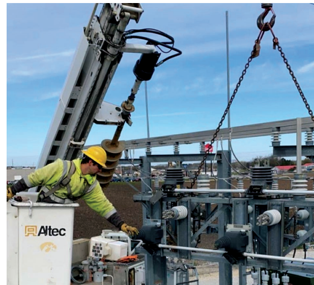
Above: Colton Dietrick working on replacing the old 600-amp switch at the Sumner substation. Below: The new 1,200-amp switch was installed in late April. Photos by: Brian Reidy
