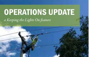
STORMS: Following a late-August storm, a tree fell into ECI REC's distribution line east of Rowley, causing it to burn down. Crews were dispatched. Because the line fell in a private right of way, Lineworker Grover had to climb the pole to put the line back up.
